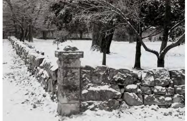
Winona Cottage Stone Wall Mortar Less Construction
